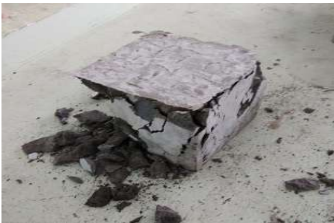
Fig 1: Failure in concrete without coconut fiber.
