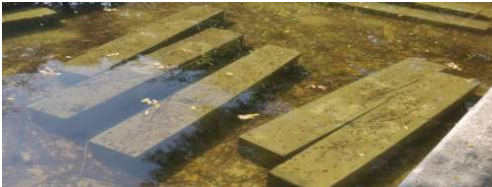
Fig 4 Immersion curing of beams
