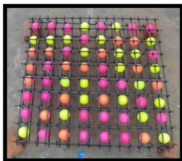
Fig - 3: Reinforcement details of Bubble Deck Slab
