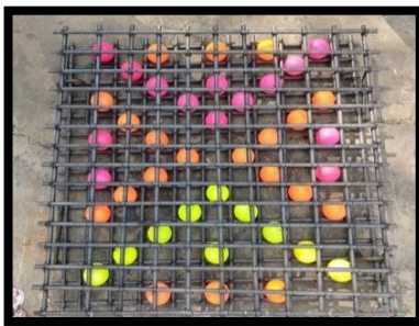
Fig - 2: Reinforcement details of Bubble Deck Slab
