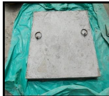
Fig - 5: Demoulding
