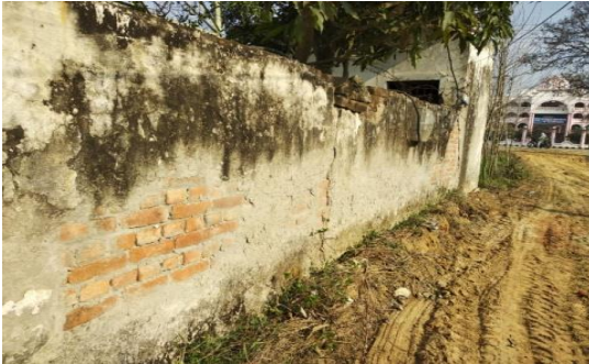
Fig 6- Plaster Decay
