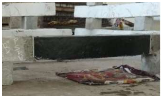
Fig-3: Beam Specimen After Retrofitting
