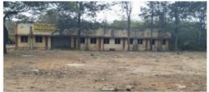
Fig.1 Hennur sewage pump
