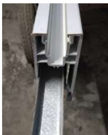
Fig -6: UPVC Frame With Hurricane Bar
