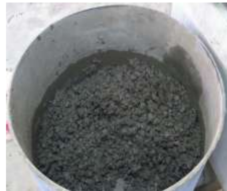
FIGURE VII. MIXING OF CONCRETE
