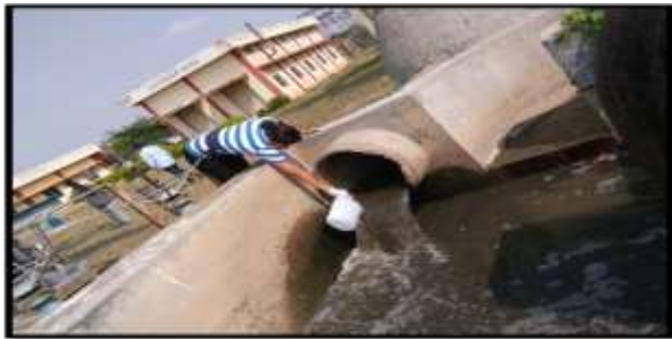
Fig-1: Sample Collection at Kesare wastewater treatment plant
