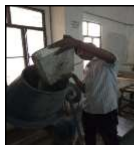
Figure-4 Mixing all material in a mixer machine.
