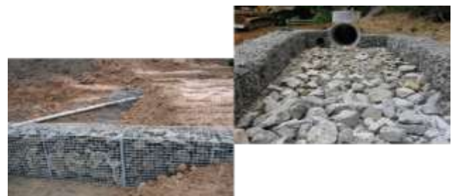
Fig.-10: Gabion wall photos
