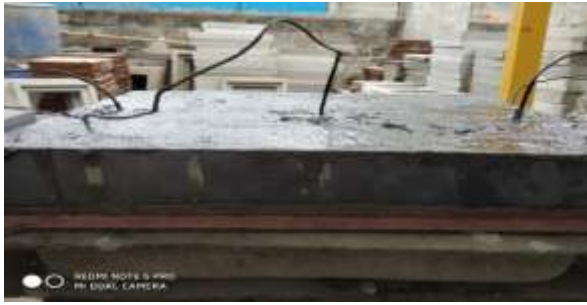
Fig: square manhole cover
