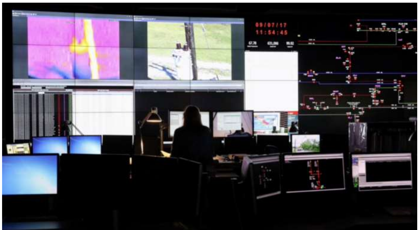
Fig. 8. Photograph of control center screens with thermal and visual drone-based video feeds being displayed.
