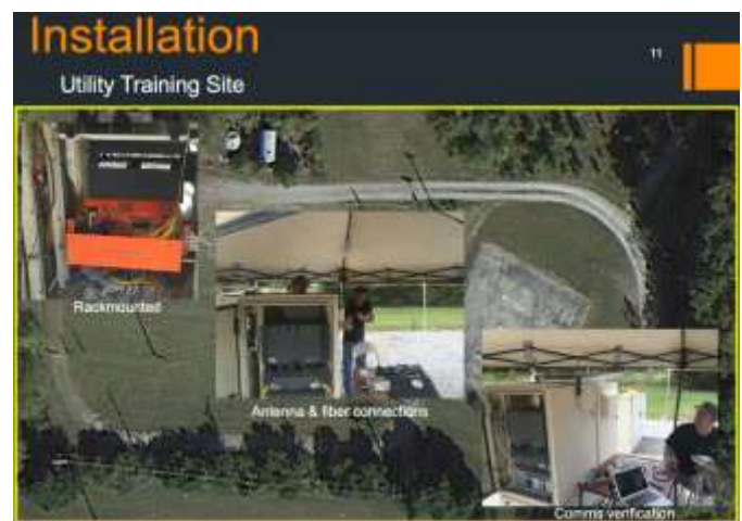
Fig. 4. Installation of the communications infrastructure at the training site.
