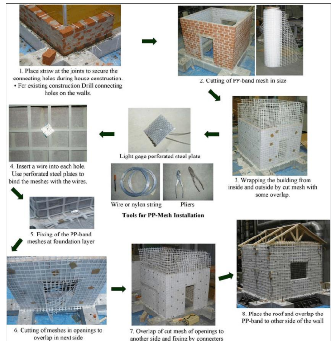
Fig. 7: PP-band mesh Retrofitting procedure for masonry house
