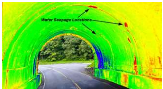
Figure 16: water seepage detection in tunnel [67]
