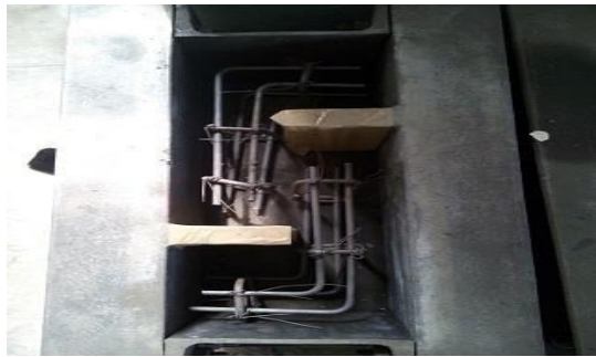
Fig 3: Reinforcement for shear specimen
