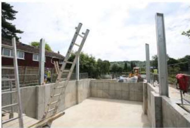
Fig - 5: Construction of amphibious house
