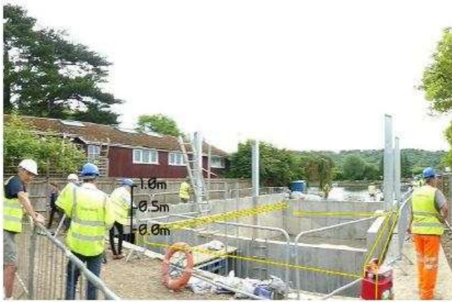
Fig - 4: Construction of amphibious house
