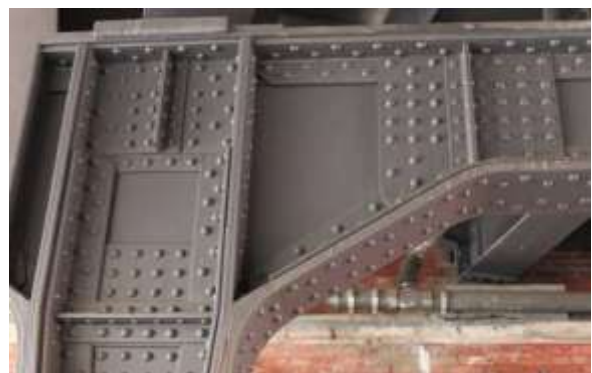
Fig: 6:Rivet joints used in railway joints
