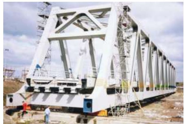
Fig5 :Sliding-in of Brinnington Bridge
