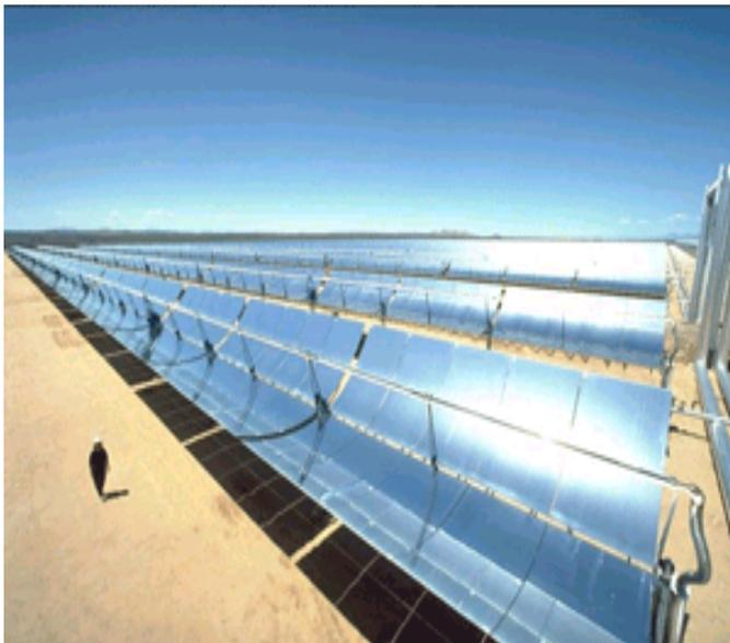
FIG 2.1. Parabolic Trough Collector
