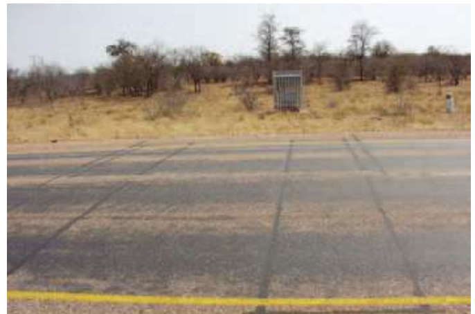
Fig:-Typical installation of inductive loops.
