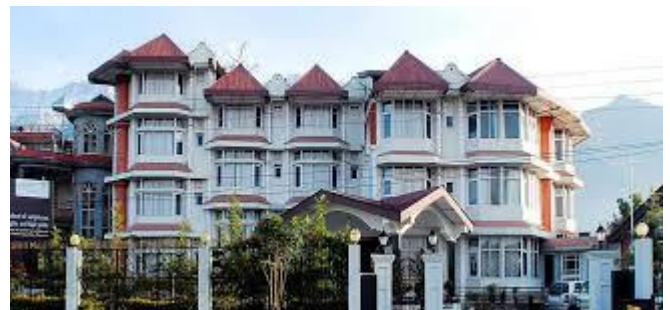
Fig -7: Typical Modern concrete building of Kangra valley
