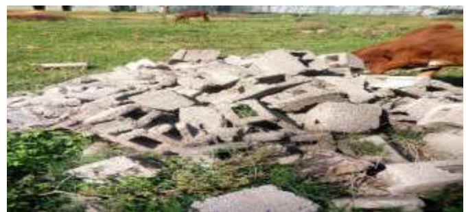
Fig 5: Poor handling HCB in building construction sites
