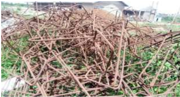
Fig 7: Wastage of steel reinforcement
