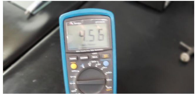
Figure 16 - RMS voltage generated by one of the phases of the hydro-generator.
