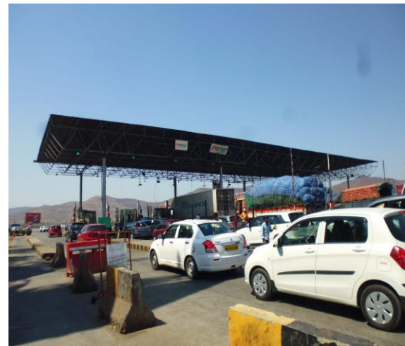
Fig -2: Lack of Display Boards at Khed-Shivapur Toll Plaza
