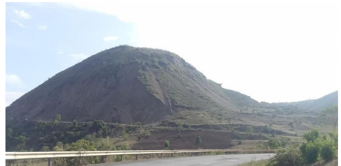
Fig -2: Photographic view of landslide from front side
