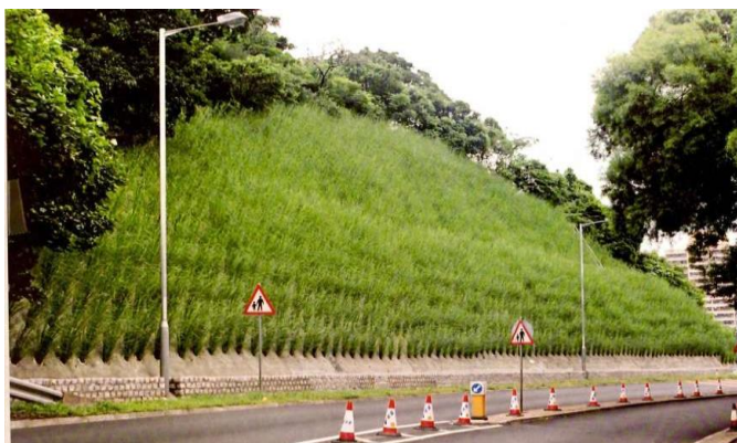
Fig -7: Vetiver Grass for Slope Protection
