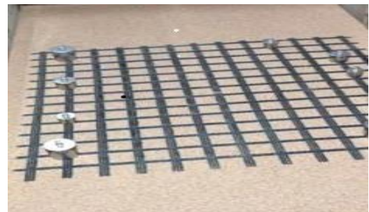
Fig 4 Placement of geogrid
