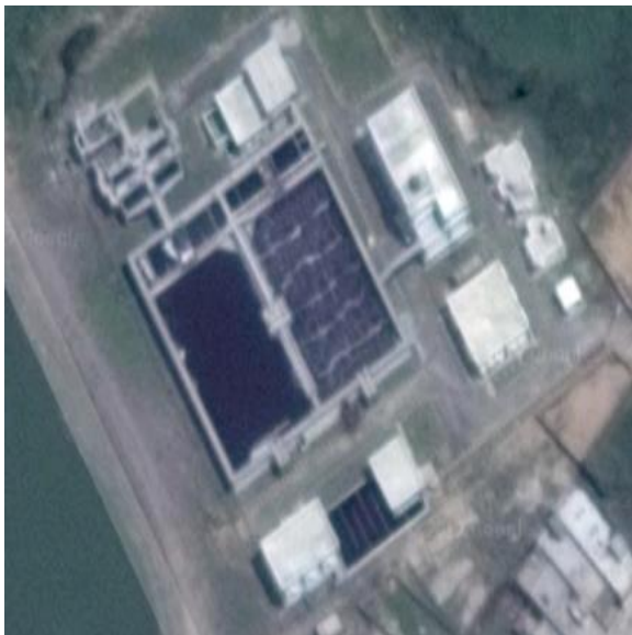
Fig.1.sewage treatment plant 15 MLD
