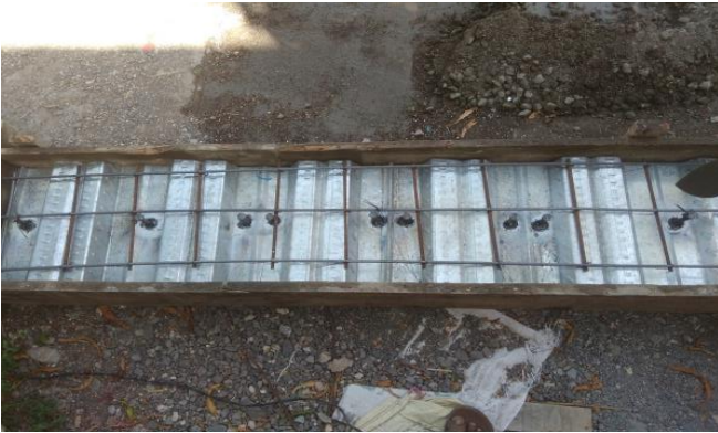
Fig.11 Reinforcement
