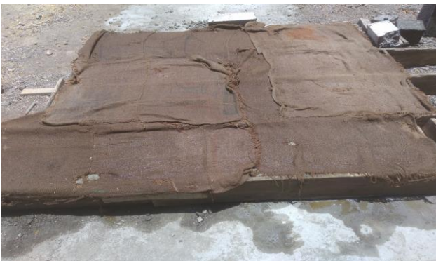
Fig.13 Curing process
