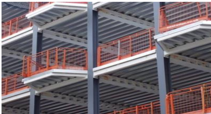
Fig.2 Composite Construction in Buildings
