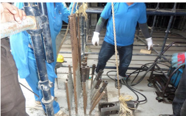
Figure joining of a coupler to Rebar
