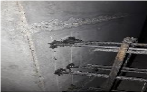
Figure: New Dowels placed
