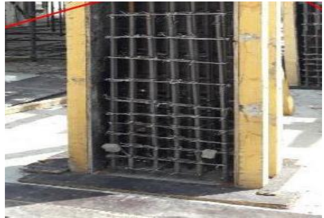
Figure: Typical Column
