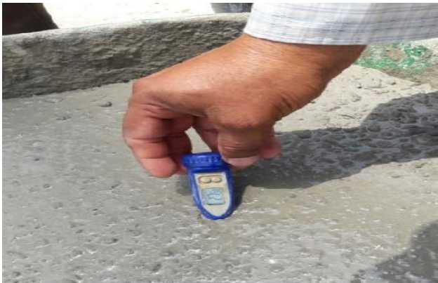
Figure: Concrete Temperature Check
