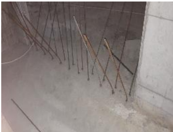
Figure: New Dowels Placed
