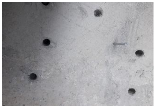
Figure: New holes drilled.
