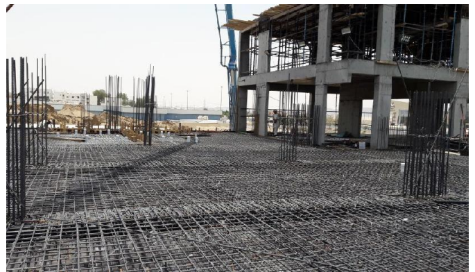
Figure: Reinforcement of Slab
