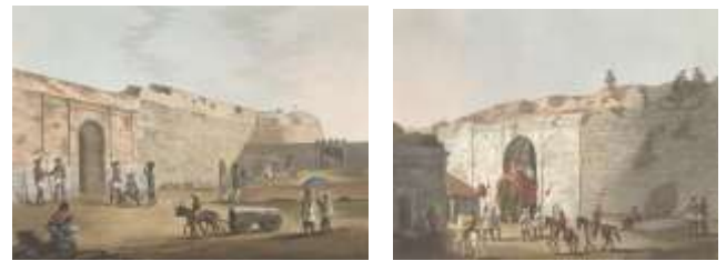
Fig. 17 & 18: Delhi gate (facing north) and Mysore gate (facing south)
