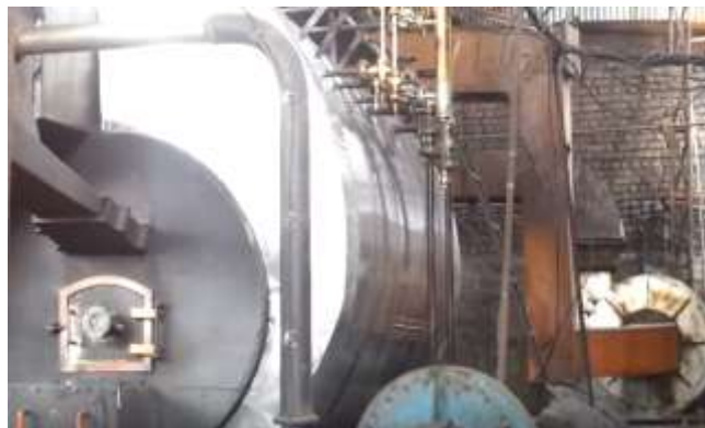
Fig - 2: Three pass fire tube Boiler
