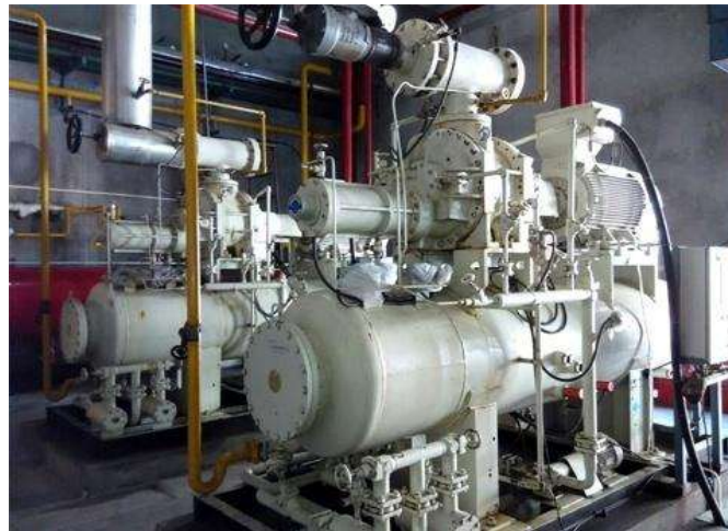
Fig -4: Single Stage Screw Type Air Compressor
