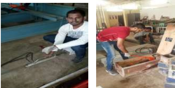
Fig 3:- Post-tensioning of beams
