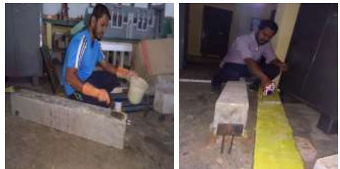
Fig 4:- Application of epoxy and aramid fibre
