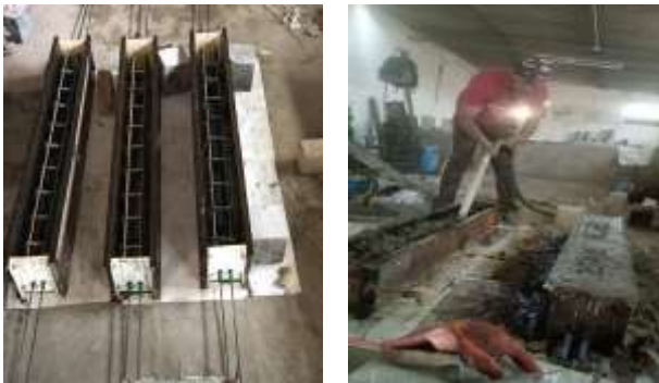
Fig 2:- Casting of Post Tensioned Beams
