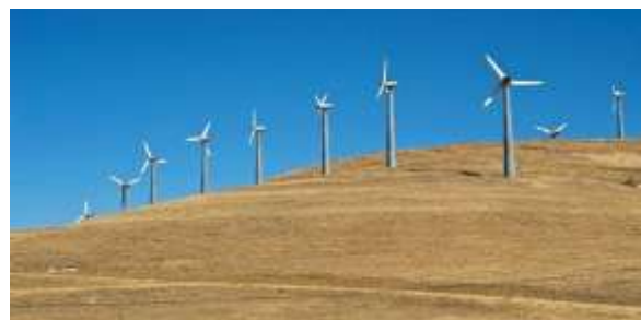
Fig -2. Wind power plant in Sindh
