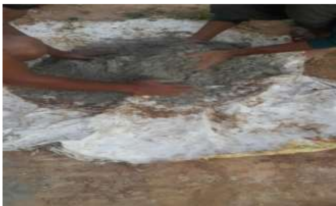
Fig-3: Dry Hand Mixing of Materials
