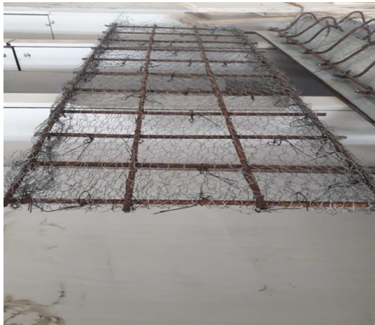
Fig-2: Flat panel with mesh reinforcement
