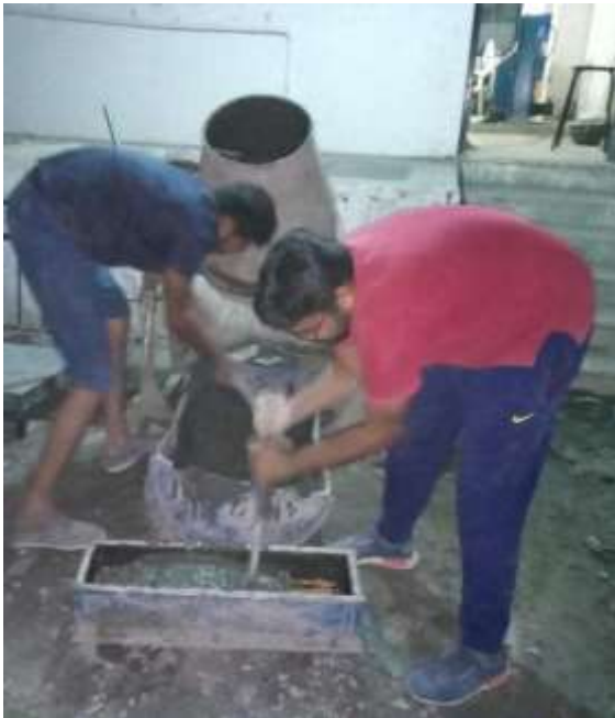
Fig-3: Casting Of Beam
