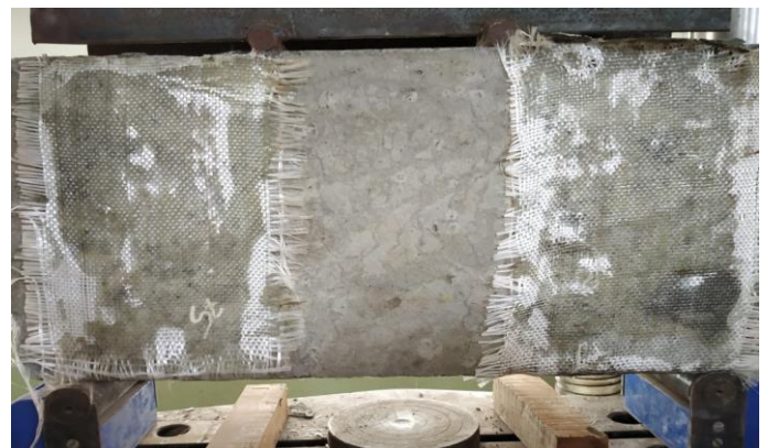
Failure and cracks on deep beam strengthened in shear
