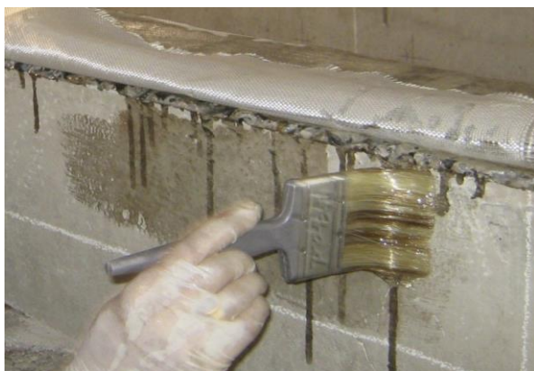
Application Of Epoxy Resin
