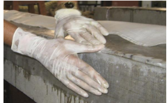
Fixing Of GFRP Plate
