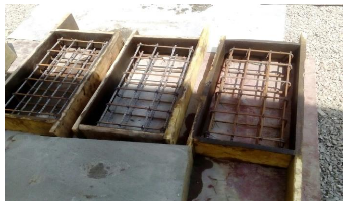
Placing of the cage in the mould
