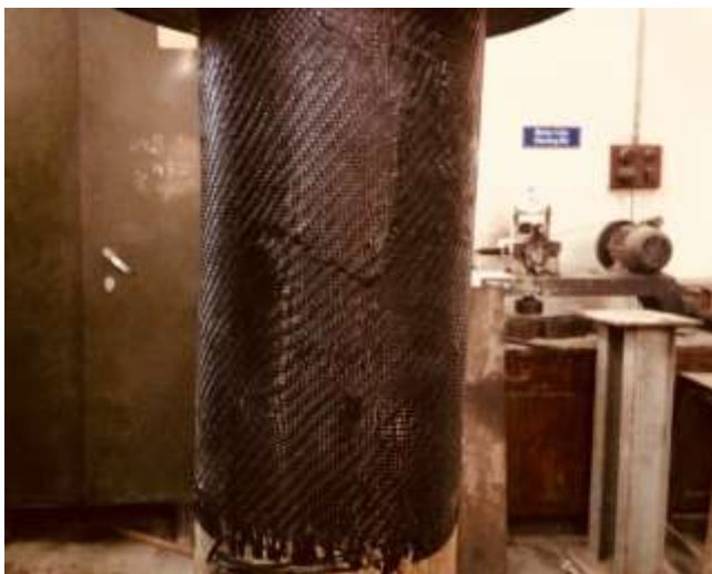
Fig. 8 Circular column with CFRP
