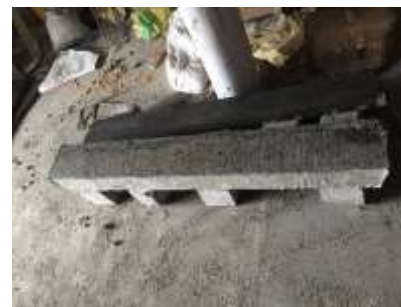
Fig -4: RCC beams
