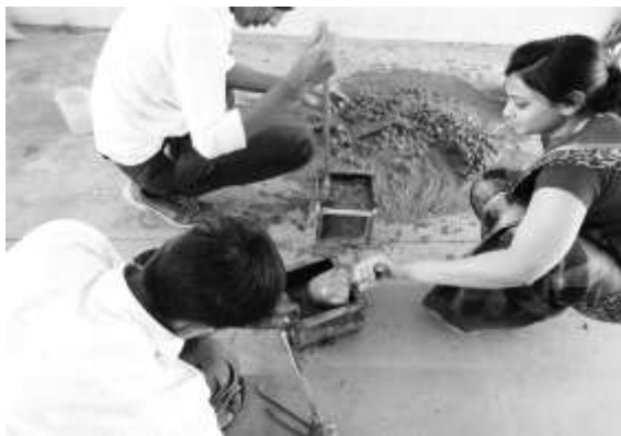
Fig.1 Mixing o concrete
