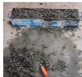
Figure 4.21: Filling the concrete into the mould
