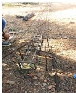
Figure 4.16: Bending of bars for beam reinforcements
