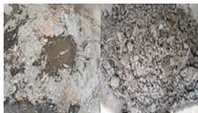
Figure 4.20: Wet mixing of materials
