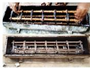
Figure 4.18: Placing of reinforcements into the moulds
