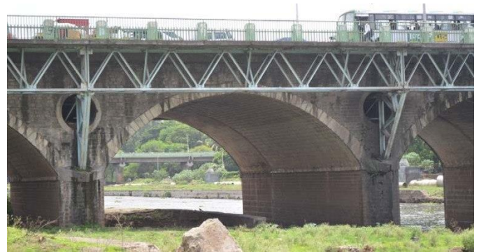
Fig -1: Sambhaji Bridge.
