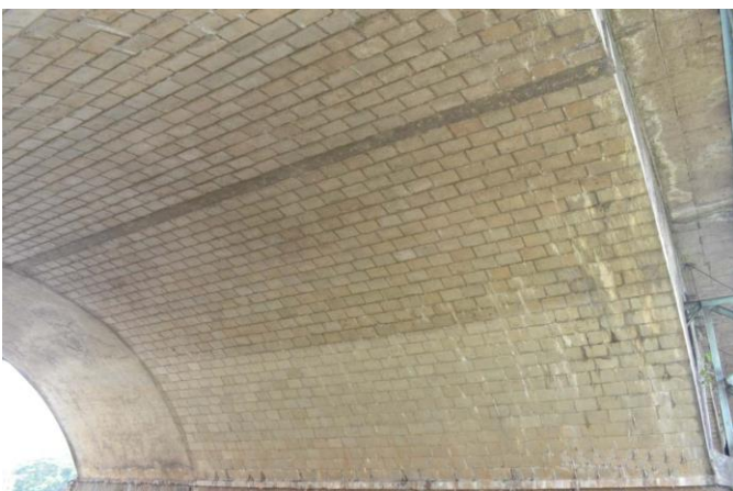
Fig -4: Arch ring with excellent stone masonry and widening by R.C.C.
