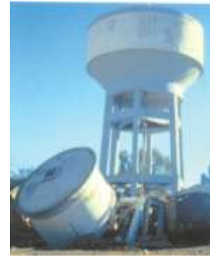
Fig -7: Failure of the reinforced concrete supporting tower of an elevated water tank during the 1980 El- Asnam earthquake, Algeria [3]
