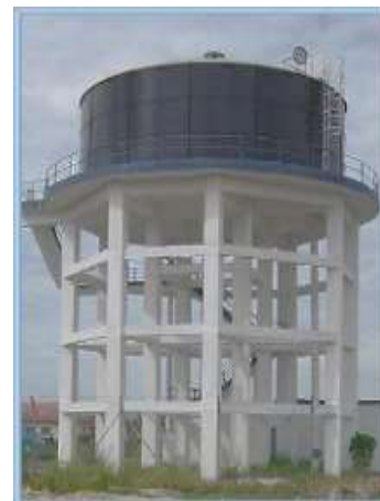
Fig -1: Elevated circular water tank with frame staging [1]
