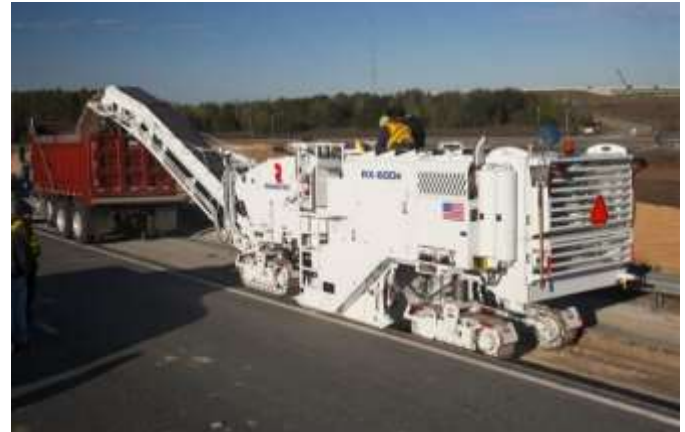
Fig 7: Rehabilitation of Bituminous pavement by milling.
