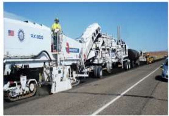
Fig -2: Hot In-place recycling (HIR)
