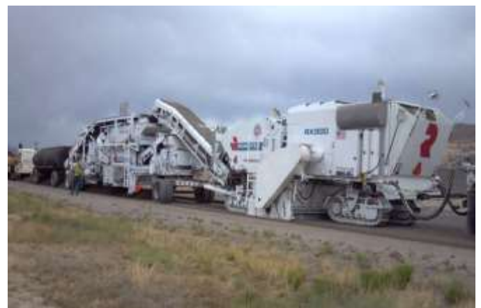
Fig -3: Cold In-place recycling (CIR)
