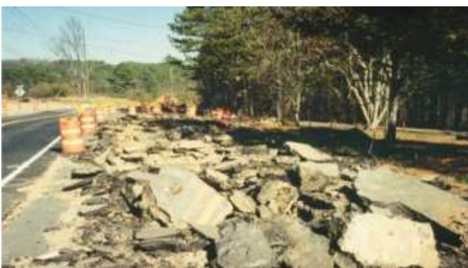
Fig -9: Full-Depth Demolition of Roadway
