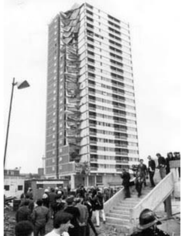
Partial collapse at Ronan Point, UK
