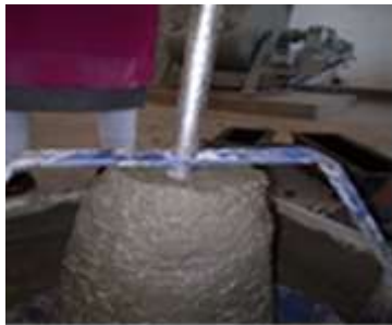
Fig-3 Slump test
