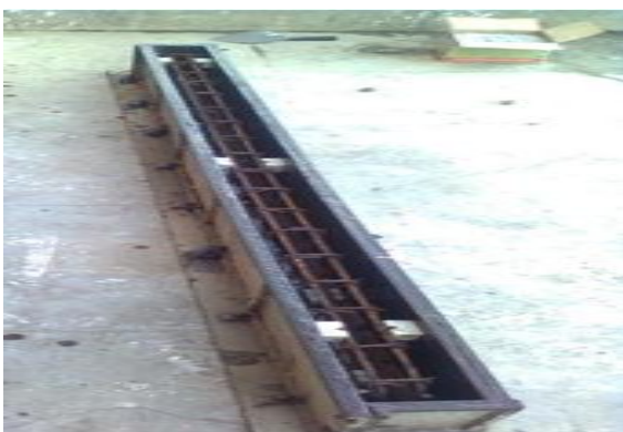
Fig -2: Casting of beam
