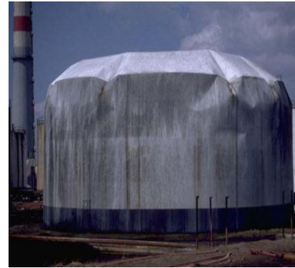
Fig -4: Roof Damage
