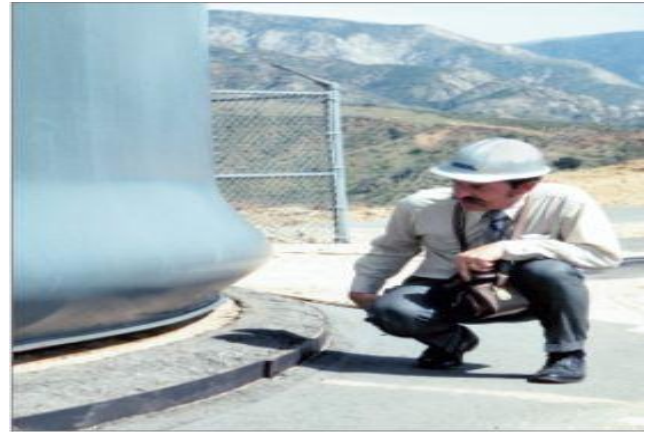
Fig -6: Elephant foot buckling
