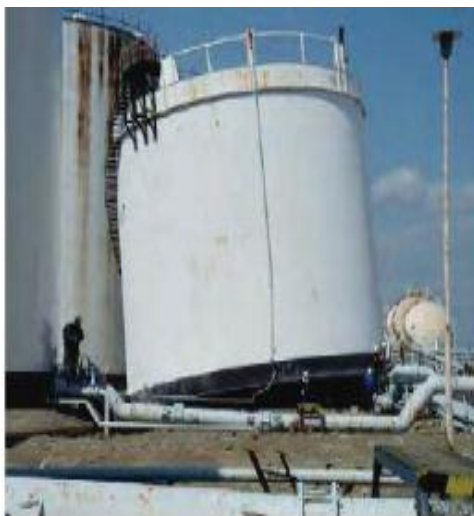
Fig -2: Uplifting Phenomenon
