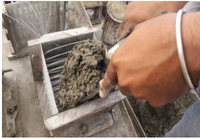
Fig [11] Pouring of concrete
