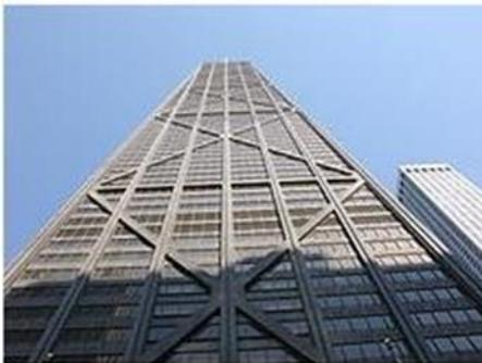
Fig-6: X Bracing
